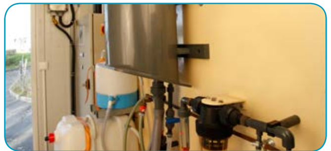
In the process: TetraCon® 700 IQ F 4 electrodes conductivity cell
